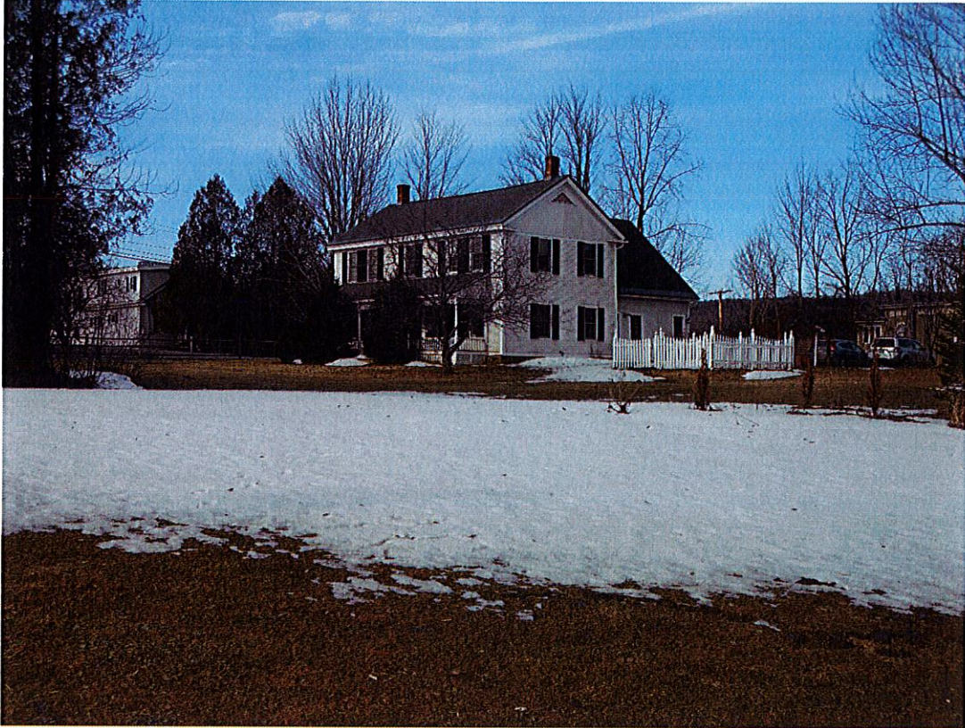
A. Photo of 40 Crosstown Road (Building 7) from Paine Turnpike (South)
