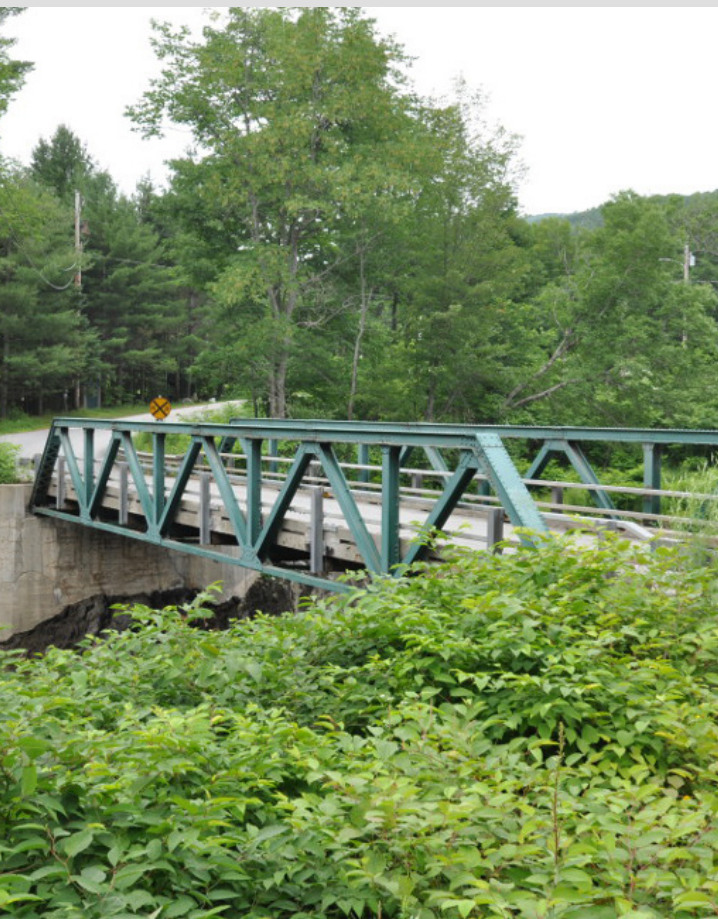
Structures Listed on the National Register The Chauncey B. Leonard house (above) on the corner of Crosstown Road and Shed Road was built in 1845 and significantly renovated in 1892. Lover's Lane Bridge (below) is a rare example of a Warren pony truss bridge. It was built in 1918 spanning the Dog River and joining Chandler Road to Route 12.
