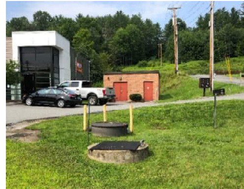
Figure 3 - Main Pump Station
