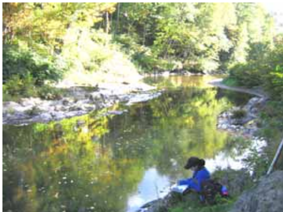
Figure 5.25: Deep pool and scour above bedrock constriction and Slaughterhouse Road Bridge
