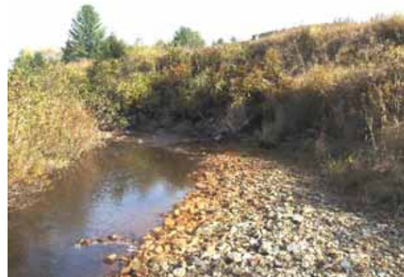
Figure 5.50: Straightened channel along railroad bed lacking riparian vegetation downstream of Rabbit Hollow Road
