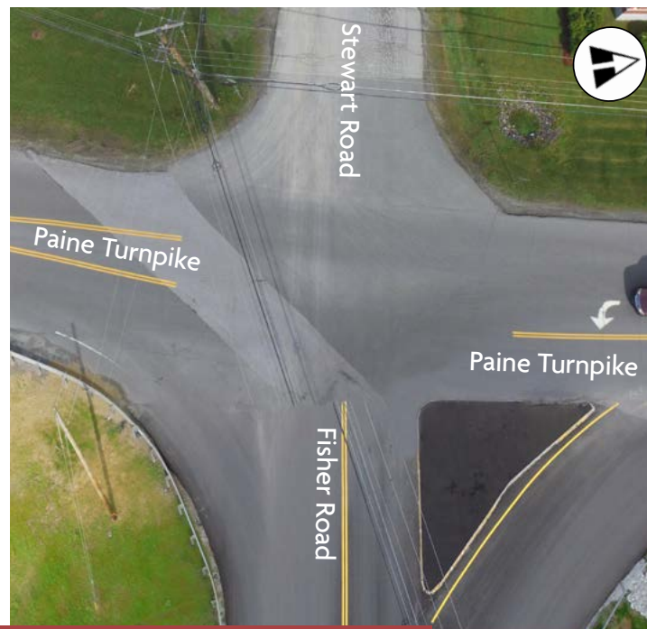
Existing Roadway Configuration
