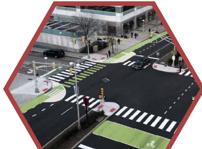
Four way pedestrian crossing improves pedestrian access throughout area.
