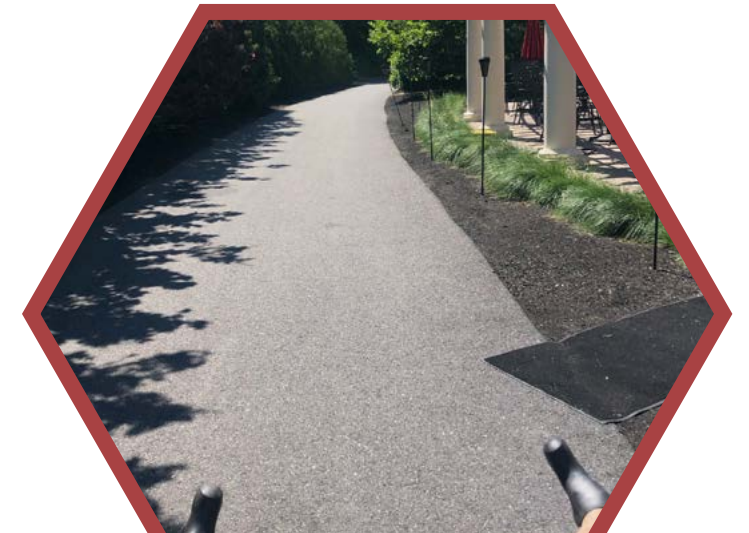
Shared Use path connects to Town Center.
