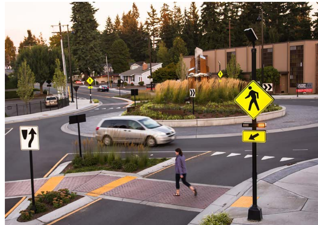
Example of roundabout in Edmonds, Washington. Note the attractive splitter island with refuge area, the rectangular rapid flashing beacons (RRFBs), brightly colored tactile warning strip and paints. Source: Carmanah Technologies Corp.
