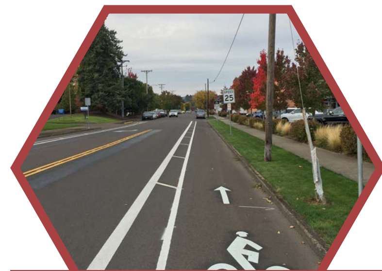
Buffered bike lanes on western side of road. Sidewalk throughout corridor to connect with shared use path.
